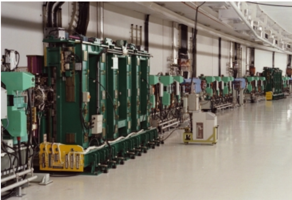
Fig. 2. One of the standard in-vacuum undulators installed in the straight section of the SPring-8 ring.
